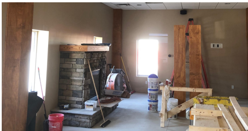
Faith of a Mustard Seed atrium under construction.
